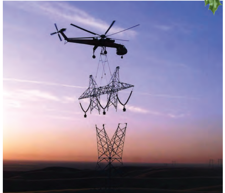
Helicopter used in construction as cranes
