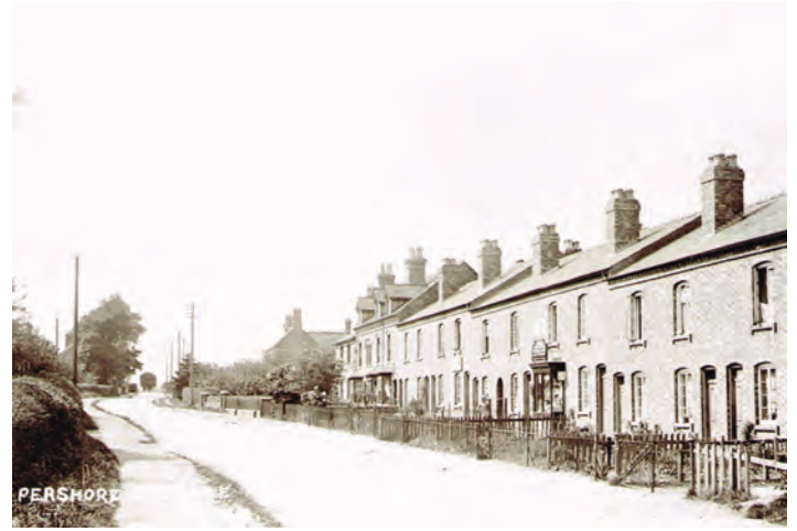
Terrace Road, Pinvin
