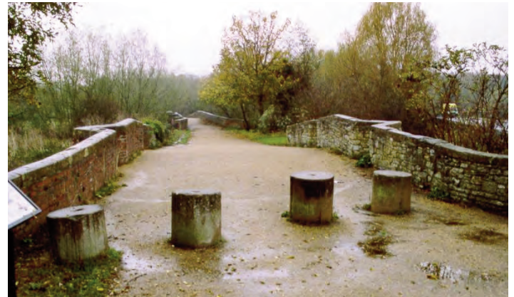
Anti-tank cylinders on the Old Pershore Bridge
